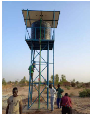
The water tower at Bendatoega being installed
